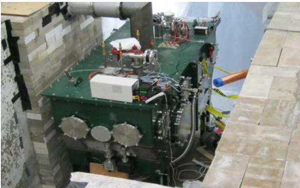
Figure 8: TDCM containing two  $\beta_0=0.53$  prototype HWR and a solenoid during installation in the test bunker.
