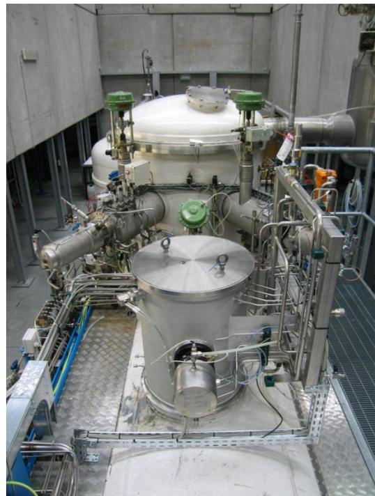
Fig. 4: Photo of ALPI Cold Box, recently upgraded with a 3<sup>rd</sup> turbine.
