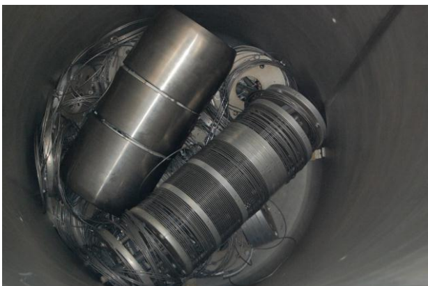
Figure 5: Collapsed accelerating column and terminal (the view from the 7th floor).
