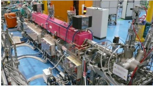
Figure 2: RFQ and IH structure in synchrotron room.
