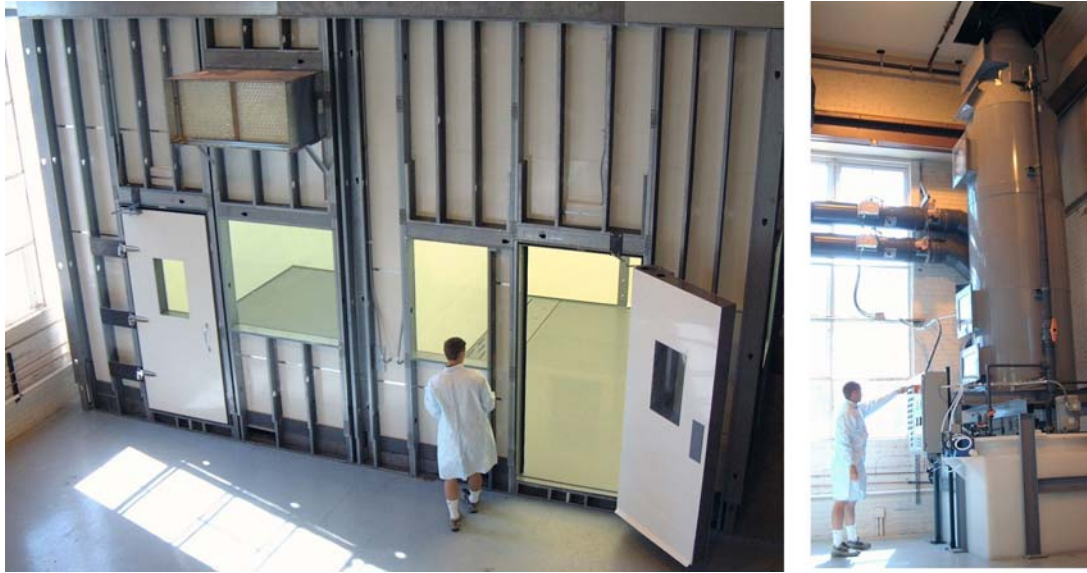
Fig. III-3. Chemical-processing rooms and a 2500 CFM air-scrubber, installed as part of a surface processing facility for superconducting cavities.
