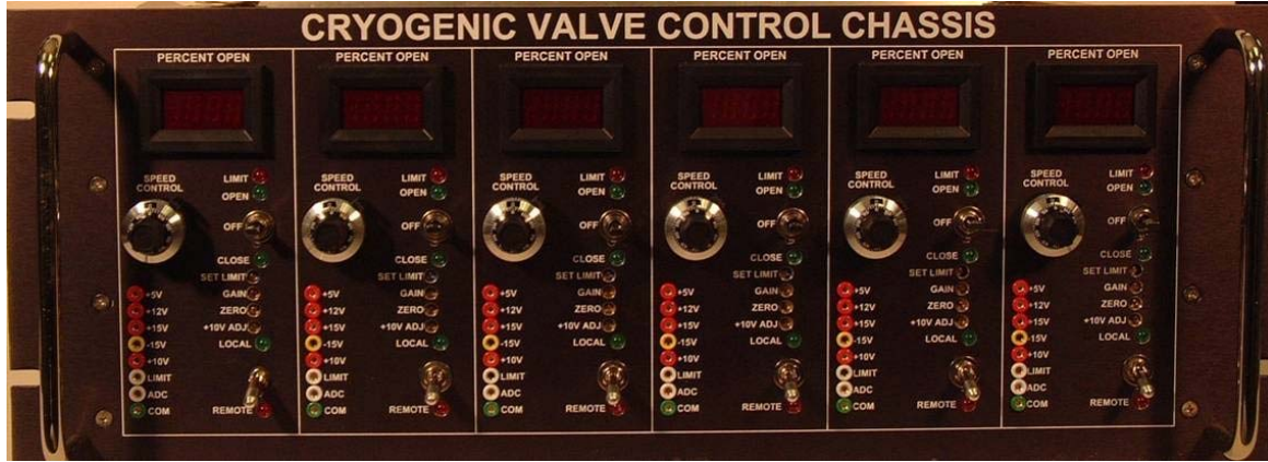
Fig. II-15. A cryogenic valve control chassis to be used to control six helium distribution valves in the ATLAS and Booster accelerating sections.
