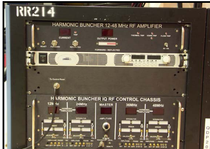
Fig. II-6. RR214 rack view showing the harmonic buncher control chassis and associated power supplies.
